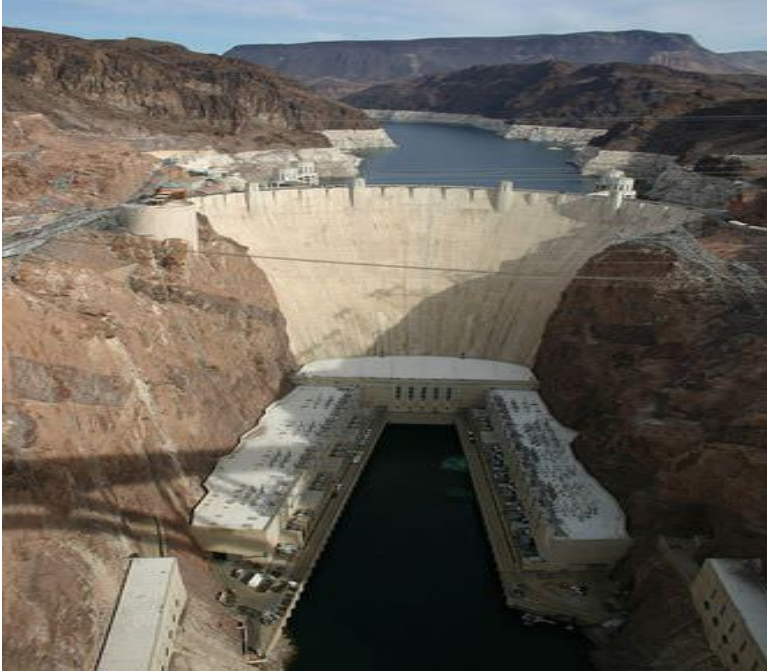
Figure 9.10 Hoover Dam, Nevada, U.S. Hoover Dam, Nevada, U.S. (credit: U.S. Bureau of Reclamation. (n.d.). Hoover Dam on the Colorado River ).
