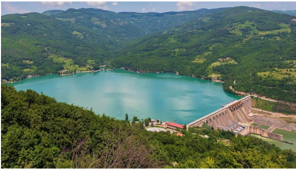
Figure 2.7 Blocked water forming a large reservoir. When blocked behind a dam, water has potential energy. (credit: Phillip / Alamy Stock Photo).
